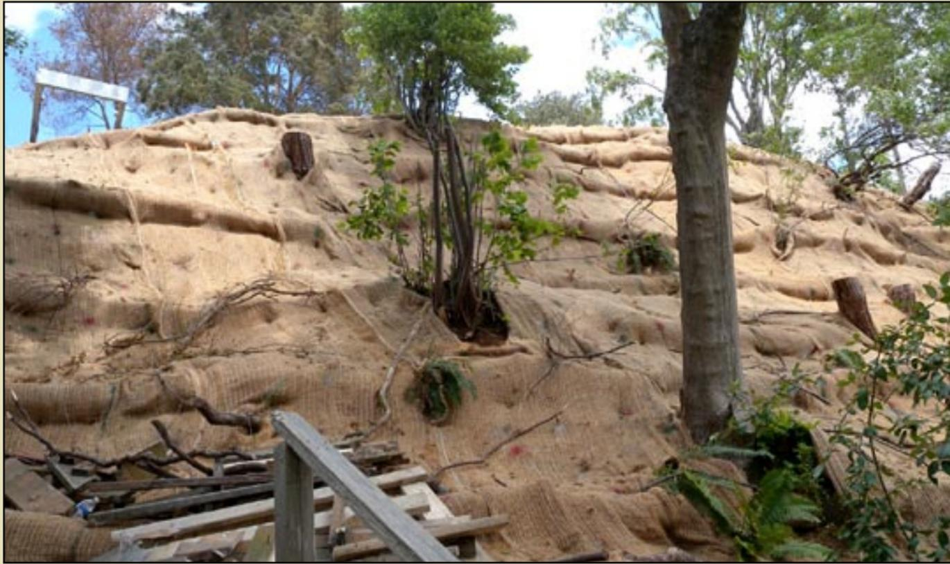
A large ivy removal and environmentally critical bank renovation in the Pacific Northwest uses geocoin for the sheet layer. Photo by Scott Baker
