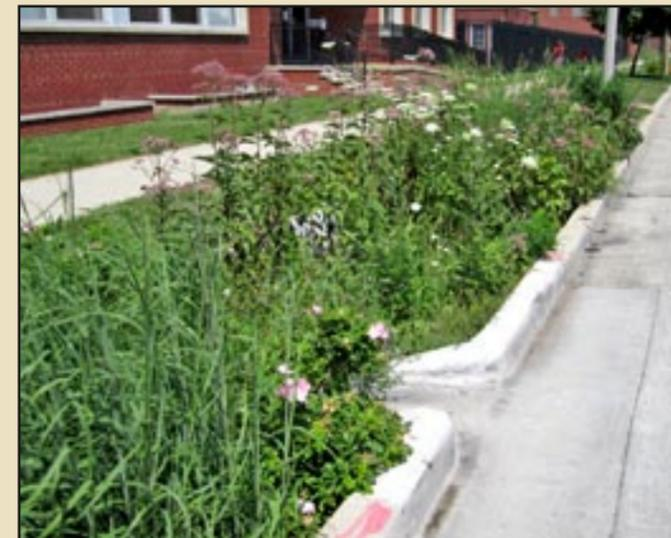
In Milwaukee, Wisconsin, runoff from the roadway enters the bioswales through curb cuts and filtrates through two layers of engineered soil and crushed stone. Photo by Scott Baran
