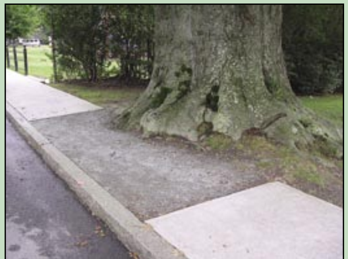
In Newport, stone dust is used to substitute for load-bearing paving slabs that often get displaced by tree roots.
