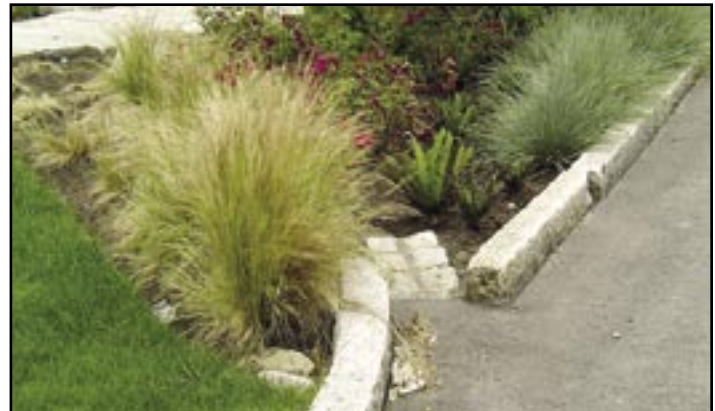
Curb openings simply but elegantly divert stormwater to plantings. photo: Ainsley Caldwell.
